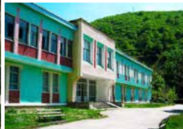
Lixha Complex, Peshkopi
